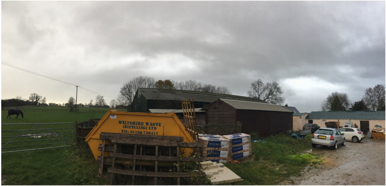
Photo 8: View looking North East Across the site
