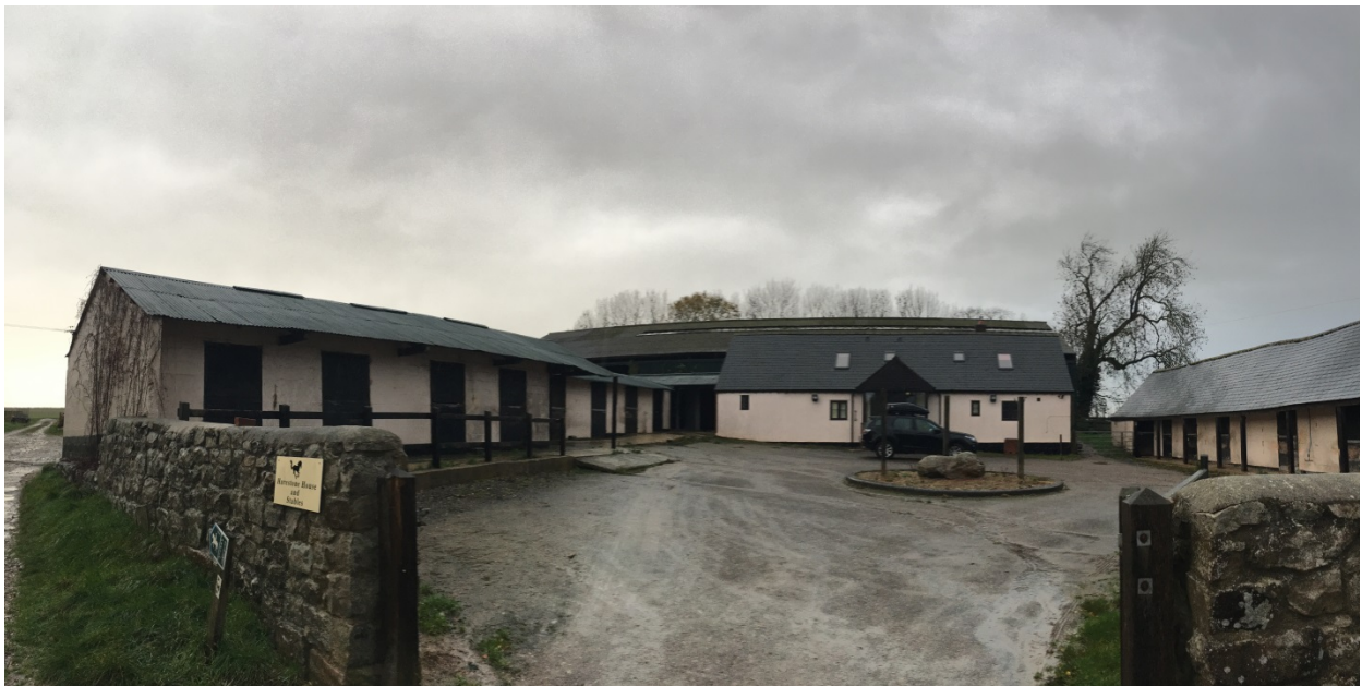
Photo 5: View of existing farm courtyard looking North West across the site
