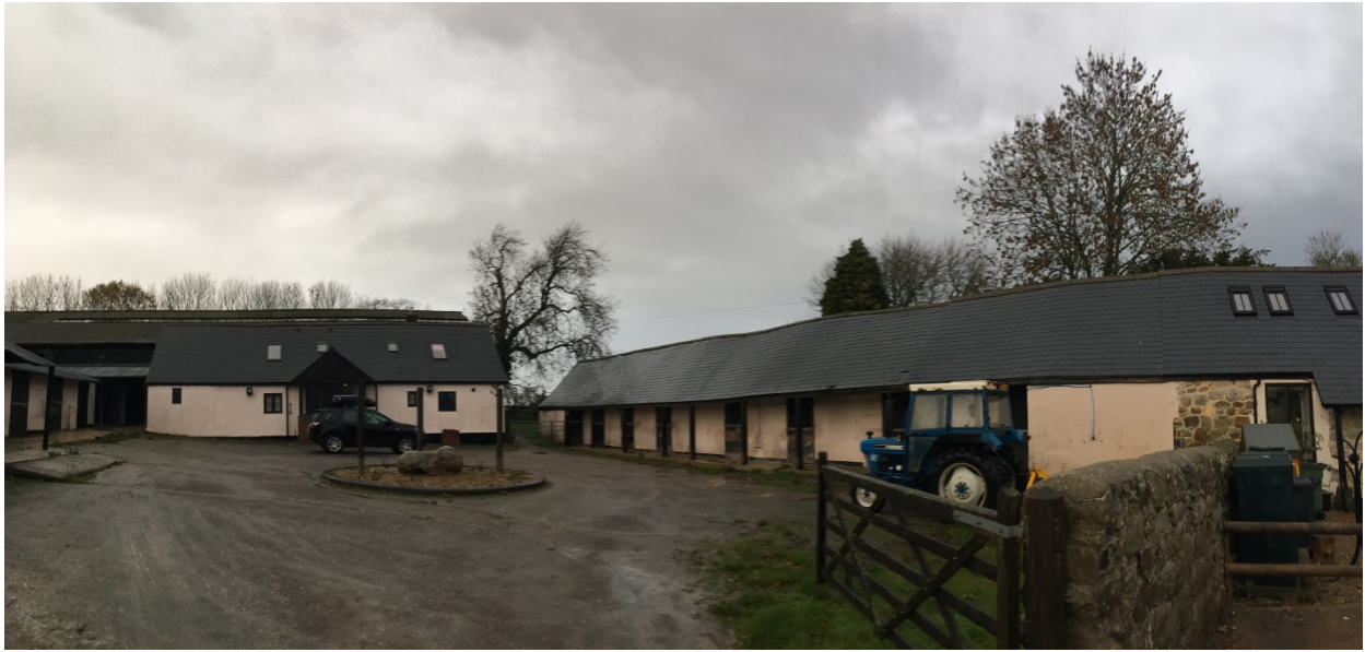
Photo 6: View of existing farm courtyard looking North East across the site
