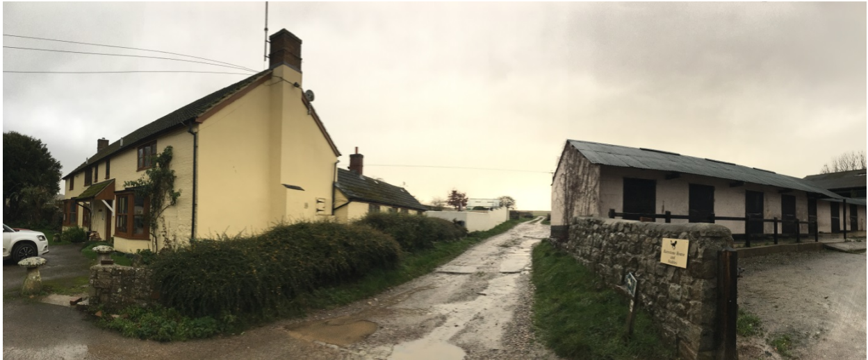
Photo 4: View from Church Lane looking South West across the site
